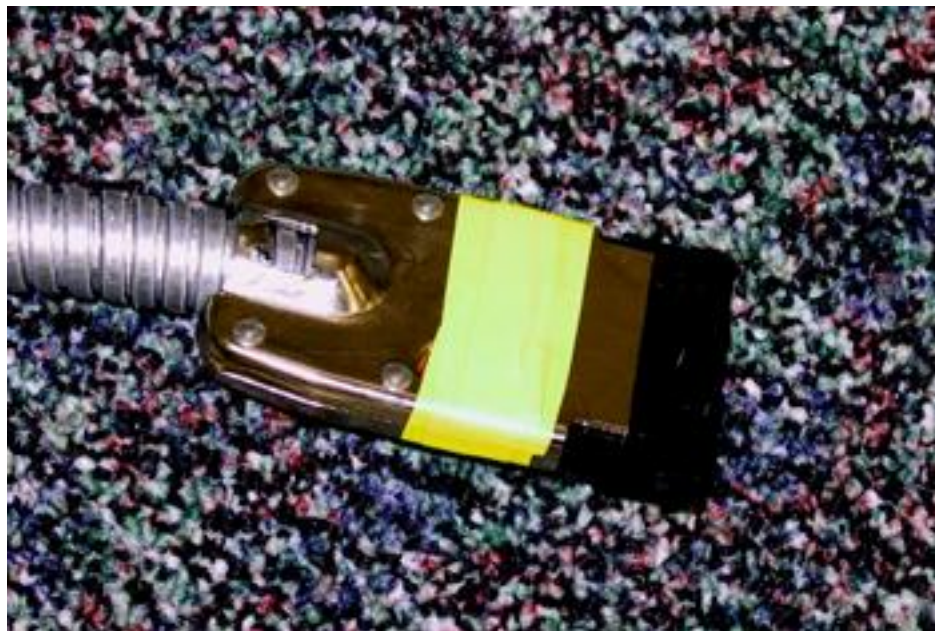
Picture 9-15 Completed Color Coding of Cable Assembly
